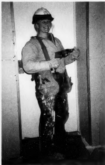
Carpenter Holly Newberry , works on renovation of the embassy.
